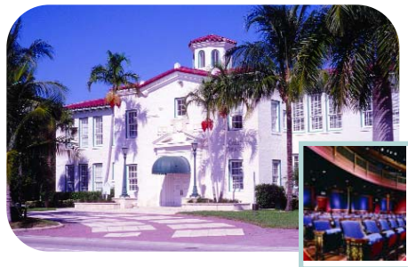
Crest Theatre (c. 1925)
